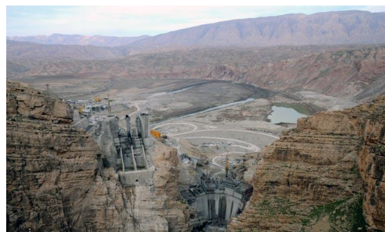
Figure 1. A view of the Seymareh dam project
